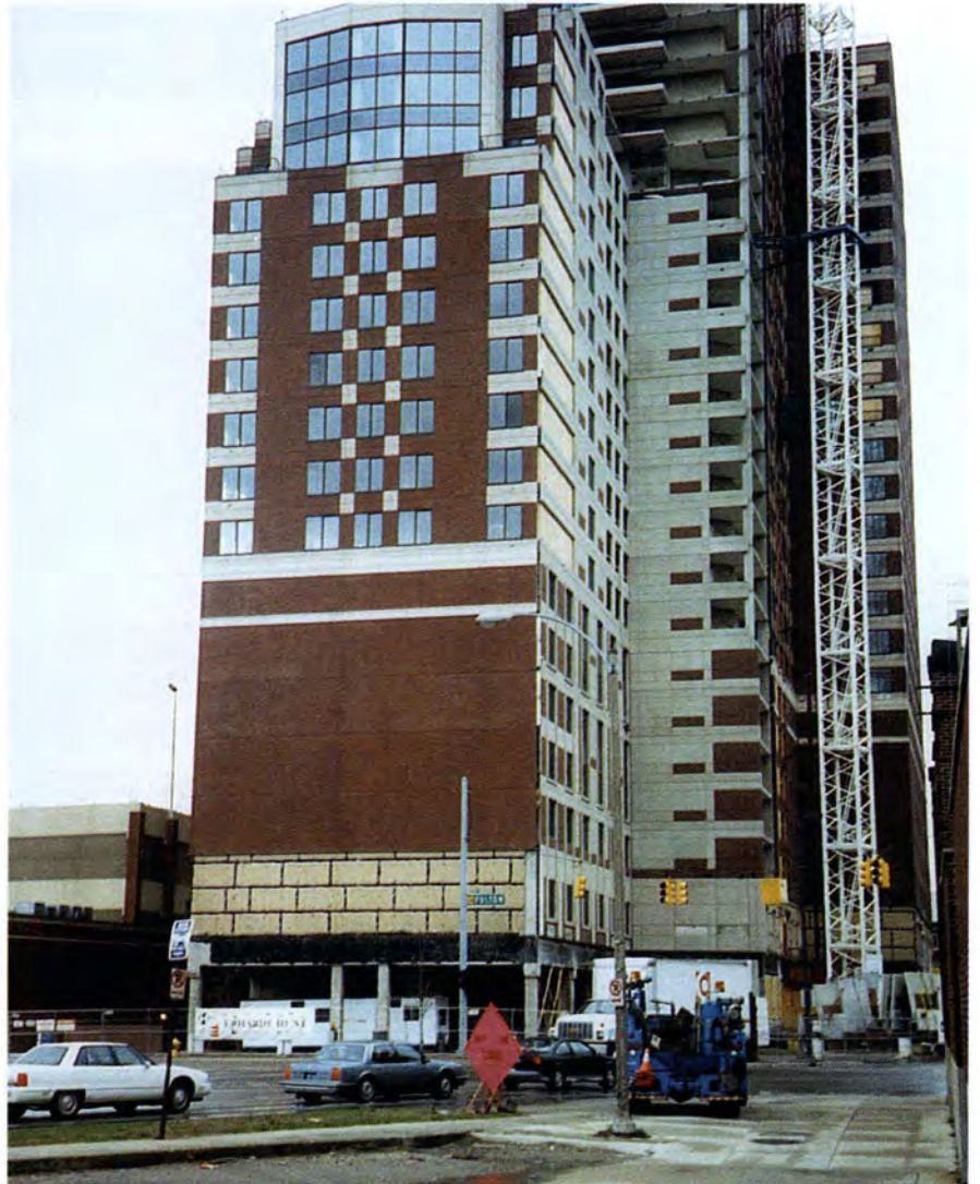
Fig. 15. Exterior view of north elevation of building showing receiving of precast components.
