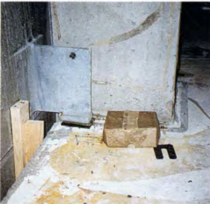
Fig. 13. Closeup of Connection #1 (see Fig. 9).
