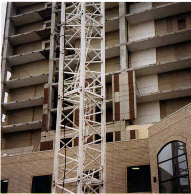
Fig. 12. Precast repair in progress.
