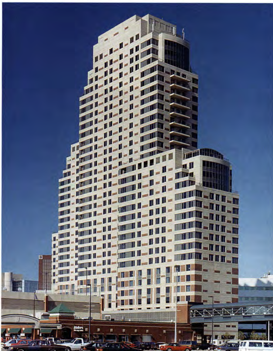
Fig. 18. Exterior view of northeast elevation of building complete with new precast cladding.
