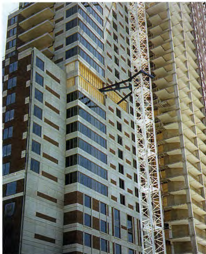
Fig. 16. Exterior view of east elevation of building showing removal of existing metal panels. Structure is ready to receive new precast panels.
