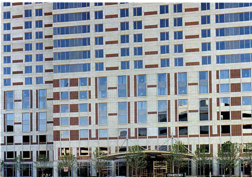
Fig. 19. Exterior view of completed east elevation of courtyard of building.
