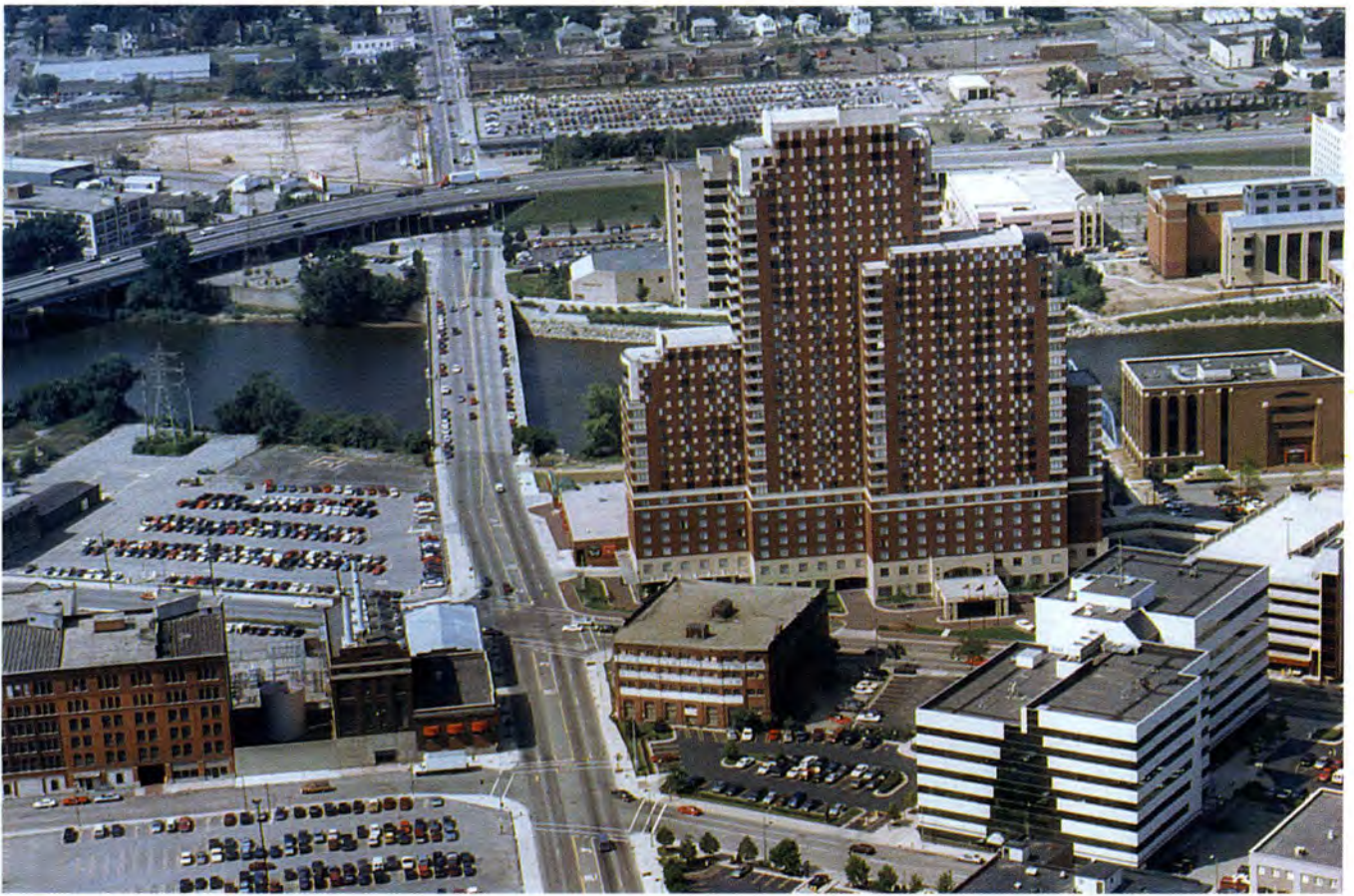
Fig. 1. Panoramic view of west elevation of Plaza Towers showing existing metal cladding.
