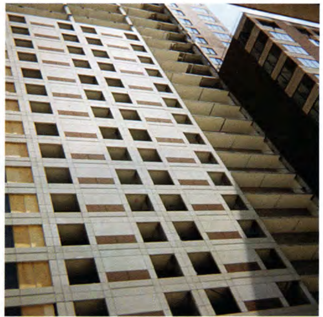
Fig. 14. Precast cladding partially in place.
