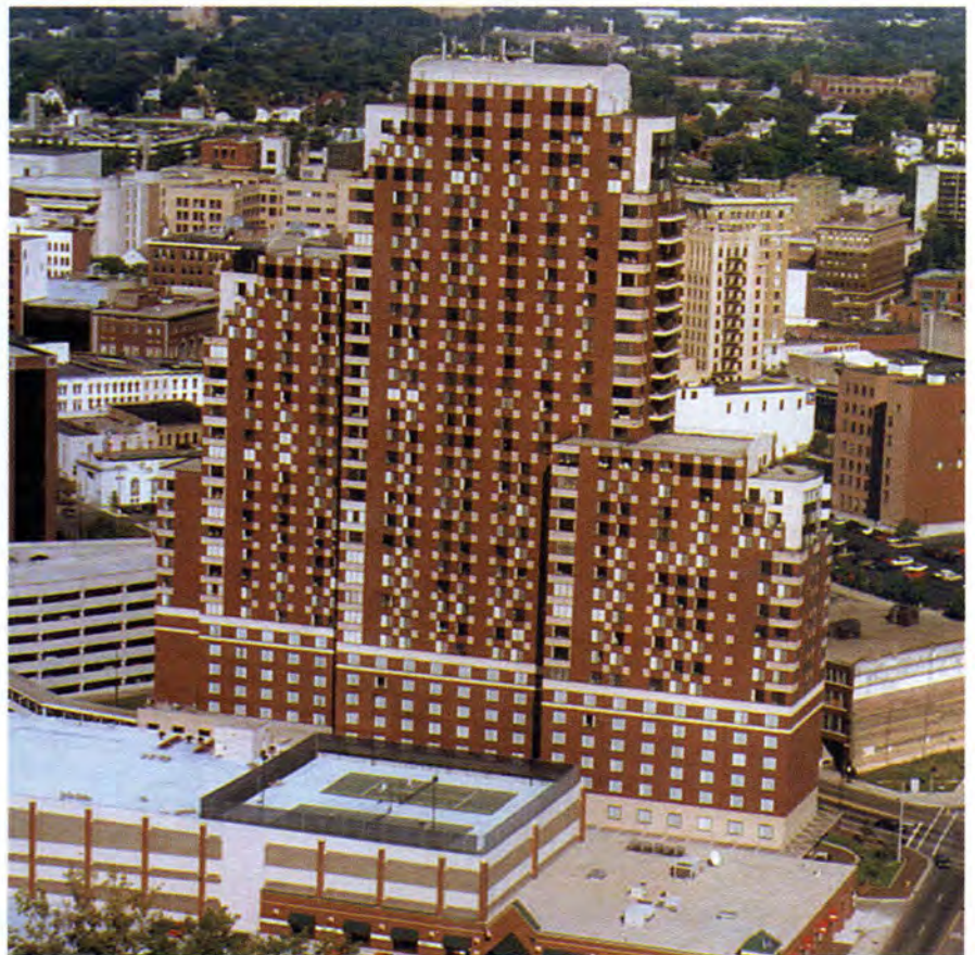
Fig. 2. Exterior view of east elevation of building showing metal cladding.
