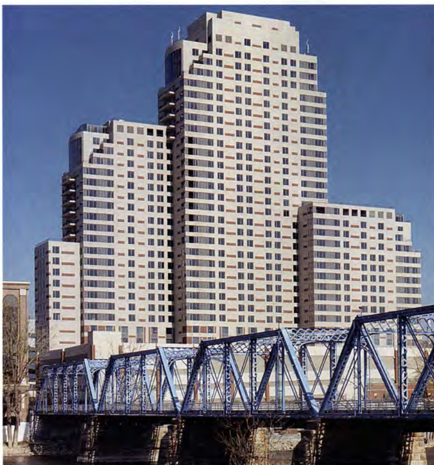
Fig. 17. Exterior view of southeast elevation of building complete with new precast cladding.
