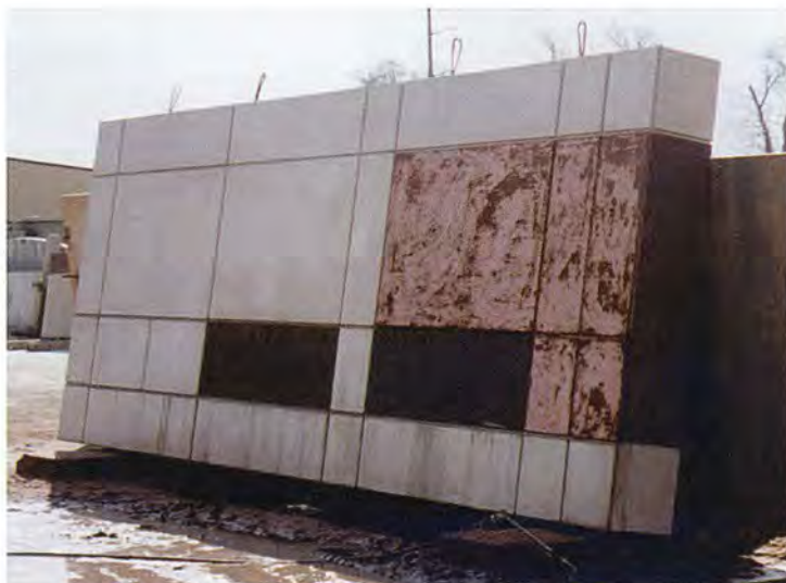
Fig. 11. Wall panel in precaster's yard.
